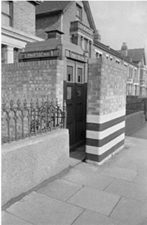
http://commons.wikimedia.org/wiki/File:Brick_blast_wall_built_to_protect_a_Police_Box_in_London,_1941_-_D2742.jpg
